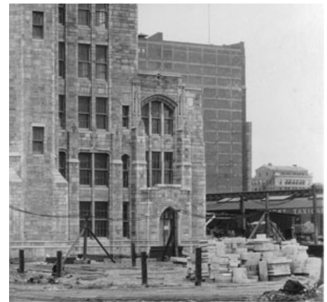
Ward Clinic Under construction, 1926
